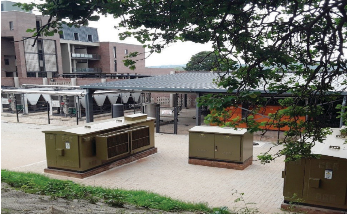
Figure 2: Chiller Plant Mini Substations with Power Factor Correction Panel
