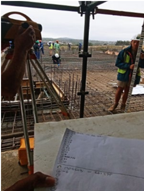
Conducting a pre-concrete survey on the slab soffit using Auto level instrument
